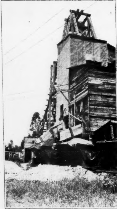
Outside Portion of Skipway Leading from Header House to Bins.
